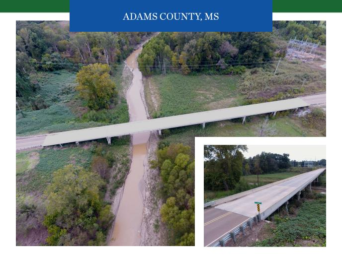
Client: Adams County Board of Supervisors Fee: \$2.33 Million Completed: 244 Working Days, 2017 This Federal Aid Project included the replacement of a bridge, 0.114 miles, and its approaches, 0.483 miles, totaling 0.597 miles.
